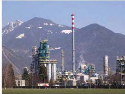
Figure 2b: the example of a modern plant
