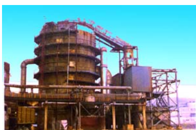
Industrial Reverse-Plant for processing of waste gases of metallurgy to H 2 SO 4 . Capacity up to 100 000 m 3 /h ("Pechenganickel" Metallurgy Plant)
